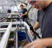
FABRICATE NEW WINDOWS
